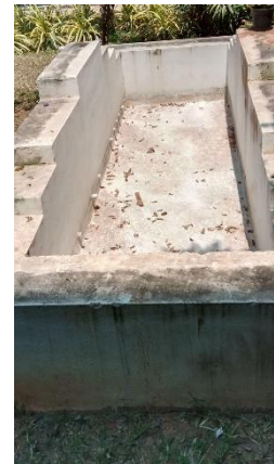
Fig. 1. Experimental site in Saveetha Engineering College
